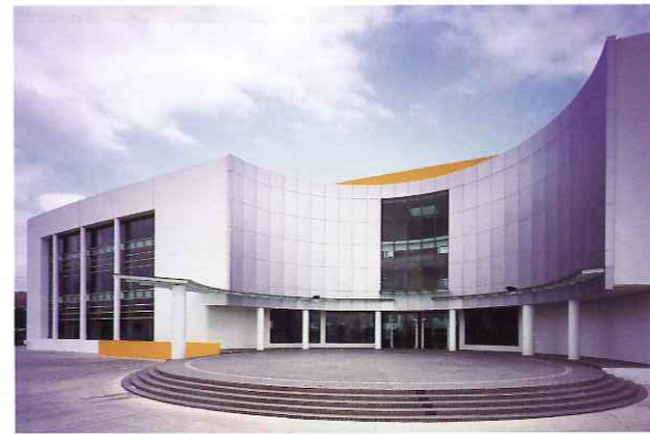
The front circular plaza. The bold textures of the spray on the walls on both sides of the plaza form a strong contrast with the smooth surface of the composite panels, enhancing the curved line, and highlighting more the entrance to the plaza. 正門圓形廣場。廣場兩邊的外牆塗有富有粗獷紋理噴漆，與復合板光滑反光的弧形牆身造成反差對比；這樣的作法更能強調弧形線條，把廣場入口突顯出來。
