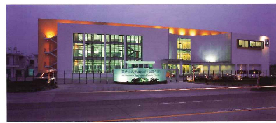
A glass curtain is fully used on the front elevation of the three-storey building for a broader view of the country scenery. A curved yellow exterior wall runs across the atrium from east to west, which covers the whole complex and forms a shining background. 建築物共有三層。大樓正面多採用玻璃幕牆，以在大樓內部可盡覽公路前的田園美景。一面黃色弧形外牆橫跨東西，越過中庭，含蓋整座建築物，遠看像一幅耀眼的背景。
